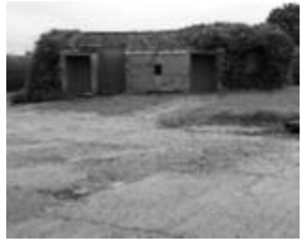
Derelict building at former RAF Downham Market
